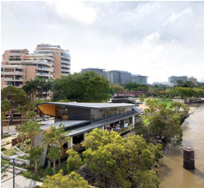
The River Quay building in Brisbane's South Bank demonstrates a number of passive design features.
