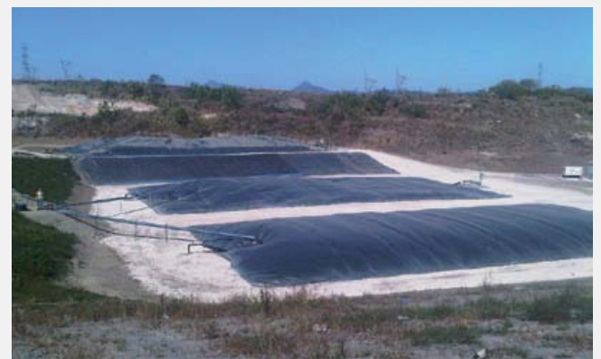
This photo shows three of the biocells at the Swanbank Renewable Energy Facility. Two contain organic waste and one contains leachates (liquid waste); the gas produced from the decay of this matter is collected by the pipes on the left of the photo.
