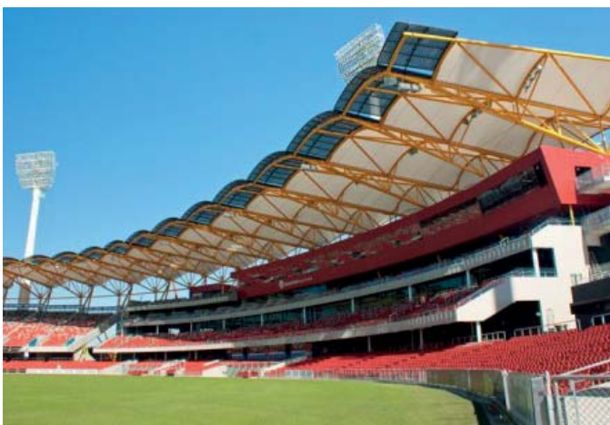
The Gold Coast's Metricon Stadium 'solar halo' provides 20% of the stadium's electricity needs.
