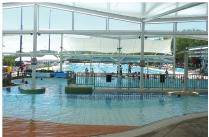
Noosa Aquatic Centre has reduced greenhouse gas emissions and costs by having more efficient pool pumping and using solar water heating.
