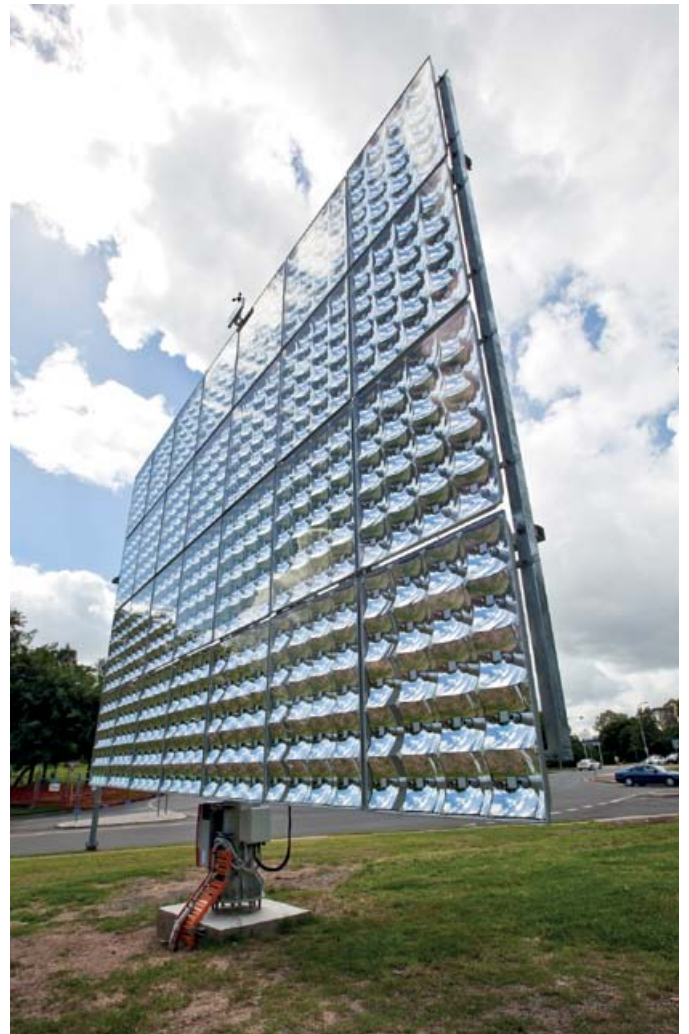
University of Queensland's ground-mounted Concentrating PV array, which tracks the sun across the sky each day.
