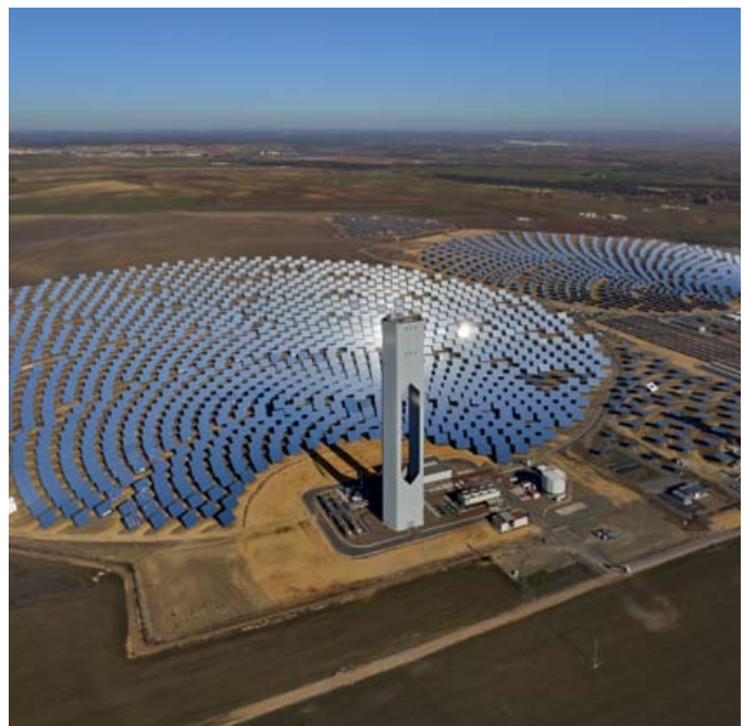
Concentrated solar thermal uses mirrors to reflect sunlight into a small area and heat fluids or salts.
